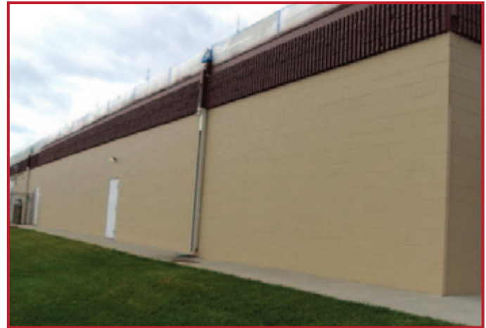
After repair and painting
